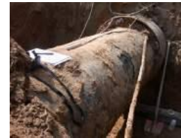
corrosion damage
