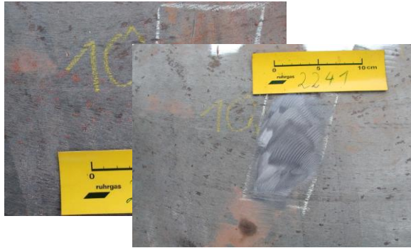
Smooth Grinding of Corrosion or Gouge
