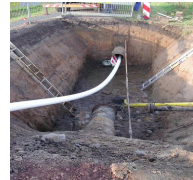
Cutting pipeline resulting in decreasing of stress/strain in coal mining areas
