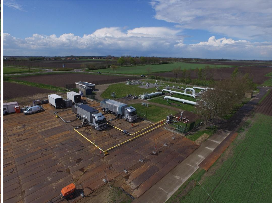
Mobile compressor (Source: Open Grid Europe, 2020)
