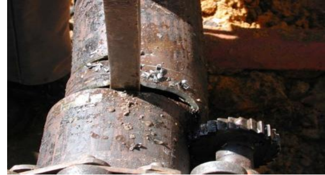
Cutting pipeline resulting in decreasing of stress/strain in coal mining areas
