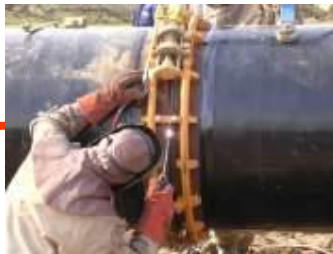
Control of • staff • welds
