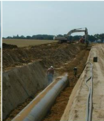
Backfilling
