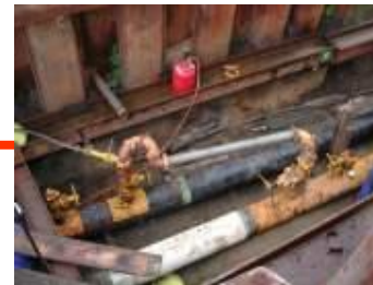
Stress testing (tightness test)
