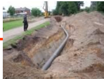
Supervision of • construction company • pipe laying
