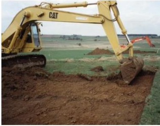
Removal of soil
