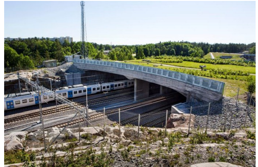
Fig. 8: wildlife bridge in Kallhäll, Stockholm (RailUK 2017)
