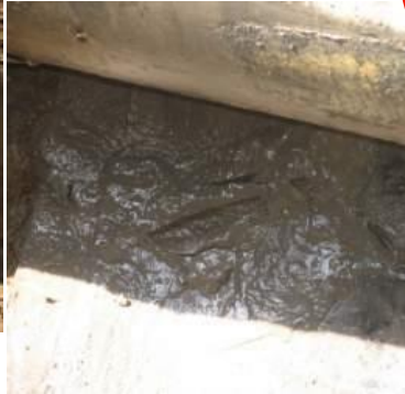
Mud in between layers
