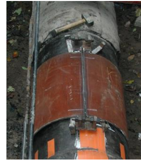
Split Sleeves with Hot Formed Ends for Repairing Large Metal Loss, Dents, Gouges
