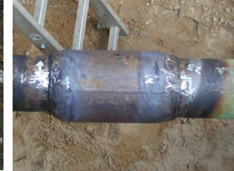
Split Sleeves with Hot Formed Ends for Repairing Large Metal Loss, Dents, Gouges
