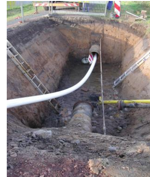
Cutting Pipeline resulting in Decreasing of Stress/Strain in Area of Coal Mining
