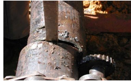
Cutting Pipeline resulting in Decreasing of Stress/Strain in Area of Coal Mining
