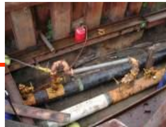
Stress testing (tightness test)
