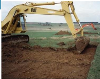
Removal of soil
