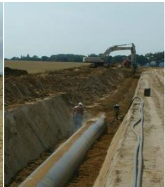
Backfilling
