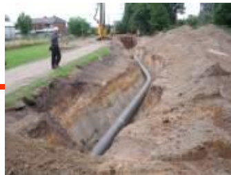
Supervision of • construction company • pipe laying
