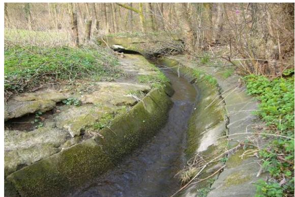
massiver Verbau: Beton
